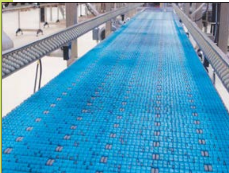
CONVEYOR FOR TRAYS WITH CANS.
